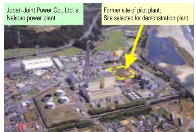
Fig. 5 Site for demonstration test. (Iwaki City, Fukushima)
